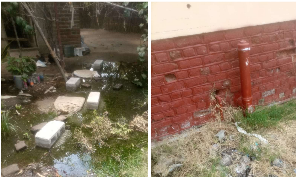
Figure 4: Broken down household septic tank (left), Dilapidated hospital sewer facility (Right)
