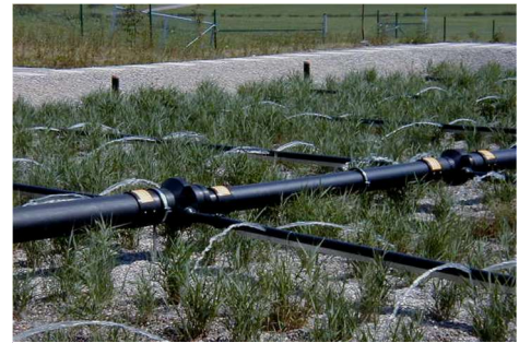
Figure 0-6: Vertical sand filter
