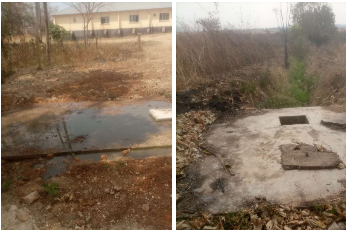
Figure 5: Overloaded hospital wastewater septic tank (left), Broken down hospital septic tank disposing untreated wastewater into the open environment (Right)
